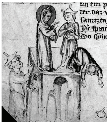
Zenon falls from the roof
